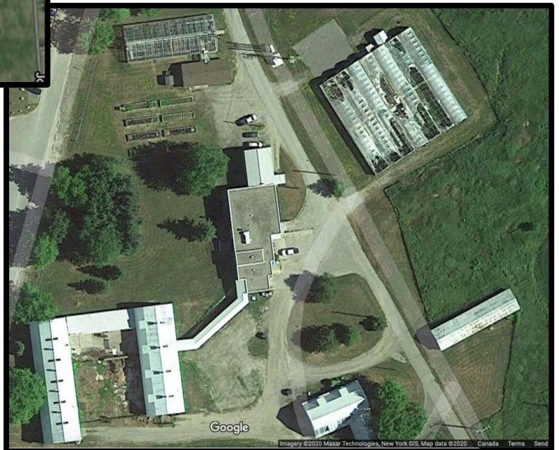
H CLOSE-UP OF THE ABATTOIR BUILDINGS AND GREENHOUSES ON THE PITTSBURGH SIDE
